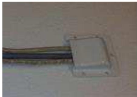
Example of cable entry plate ready to be glued and screwed into position.
